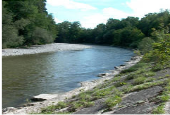
FIGURE 19: EMBANKMENT MADE IN A RIVER TO REDUCE THE INTENSITY OF FLOOD
