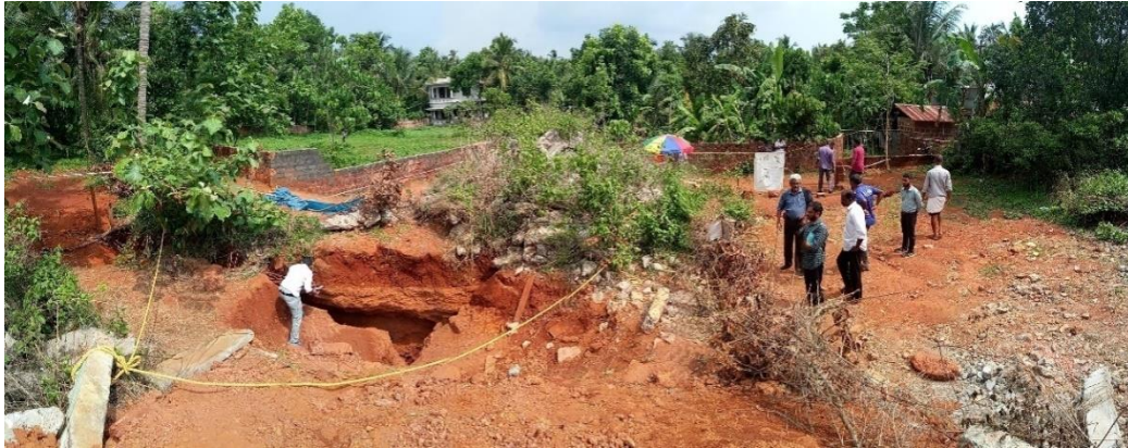
Figure 16 Ground fissure near Zainudin's house-2018
