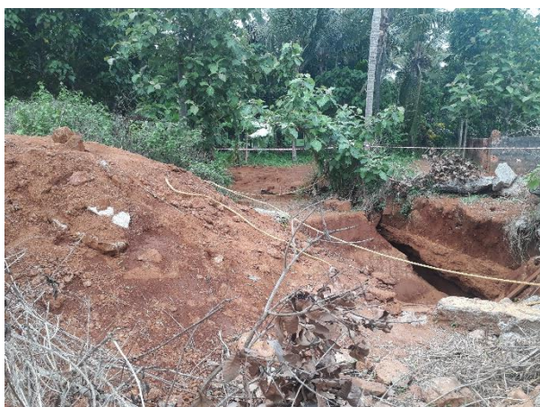
Figure 2 Fissure in Zainudin's land
