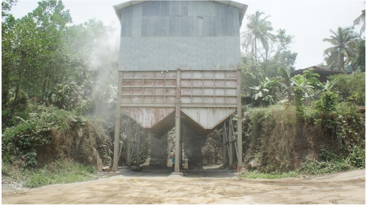
Photo 5: Stone crushing unit
