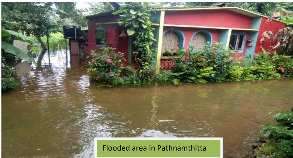
Flooded area in Pathnamthitta
