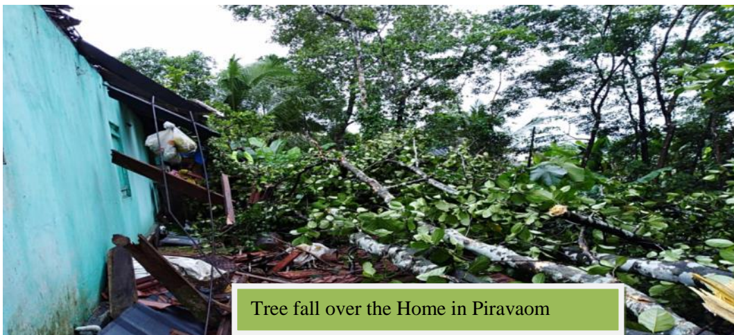
Tree fall over the Home in Piravaom
