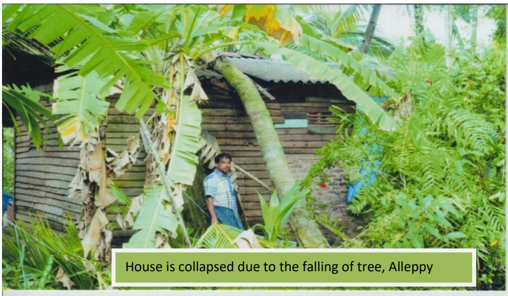
House is collapsed due to the falling of tree, Mavelikkara Allepy
