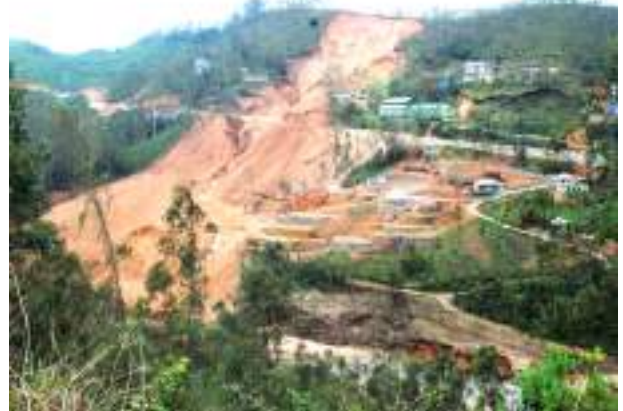
Fig.5. Landslide at Munnar Arts college in 2005 and 2018
