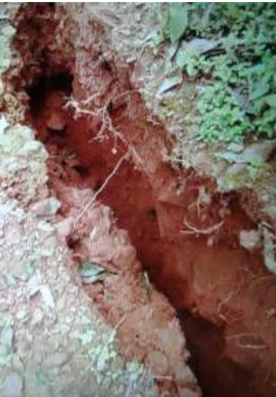
Fig.4. Slab slide occurred in Wayanad district (2018)
