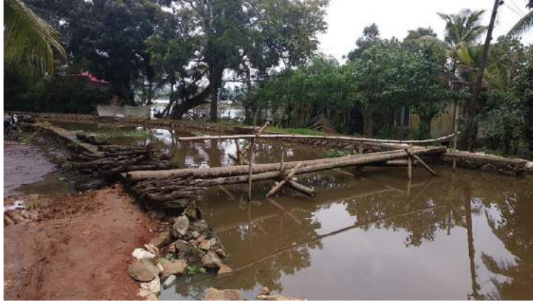
Figure 10: Temporary structure created by locals using bamboo stick which restricted the movement of boats in Ramankary
