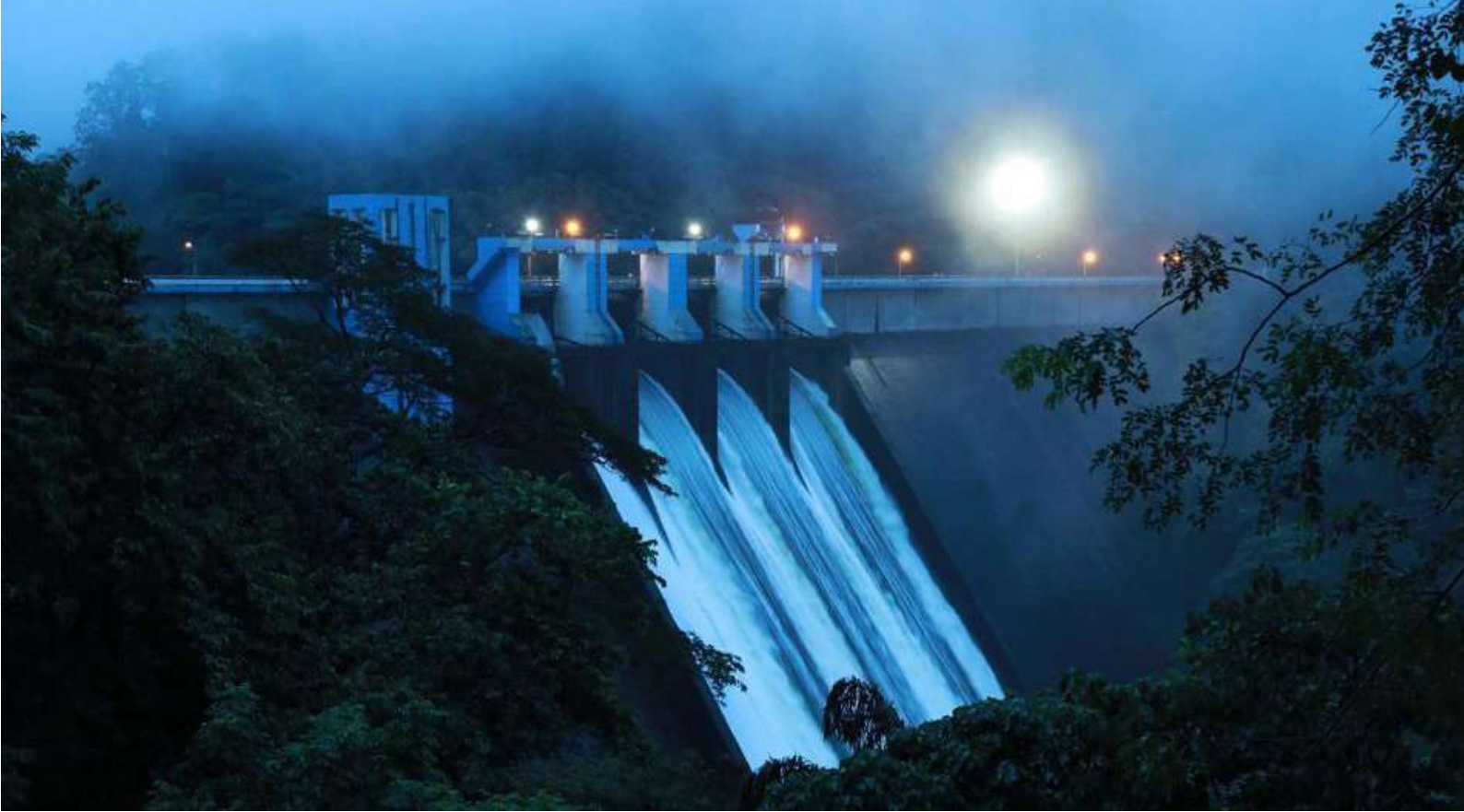
Water gushes out of Idamalayar dam as shutters of the dam opened with the storage level crossing 169 metre | AFP
