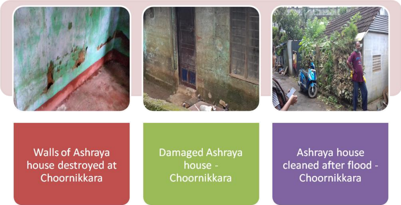
Houses of Ashraya beneficiaries at Choornikkara
