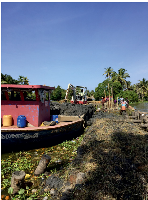
Figure 5. View of the bund reconstruction efforts that secures Kanakassery, Valiyakari, and Meenapally paddy polders from the Vembanad Lake in Kuttanad. The left of the bund is the Vembanad Lake and the right of the bund is the paddy polders that span over 750 acres.
