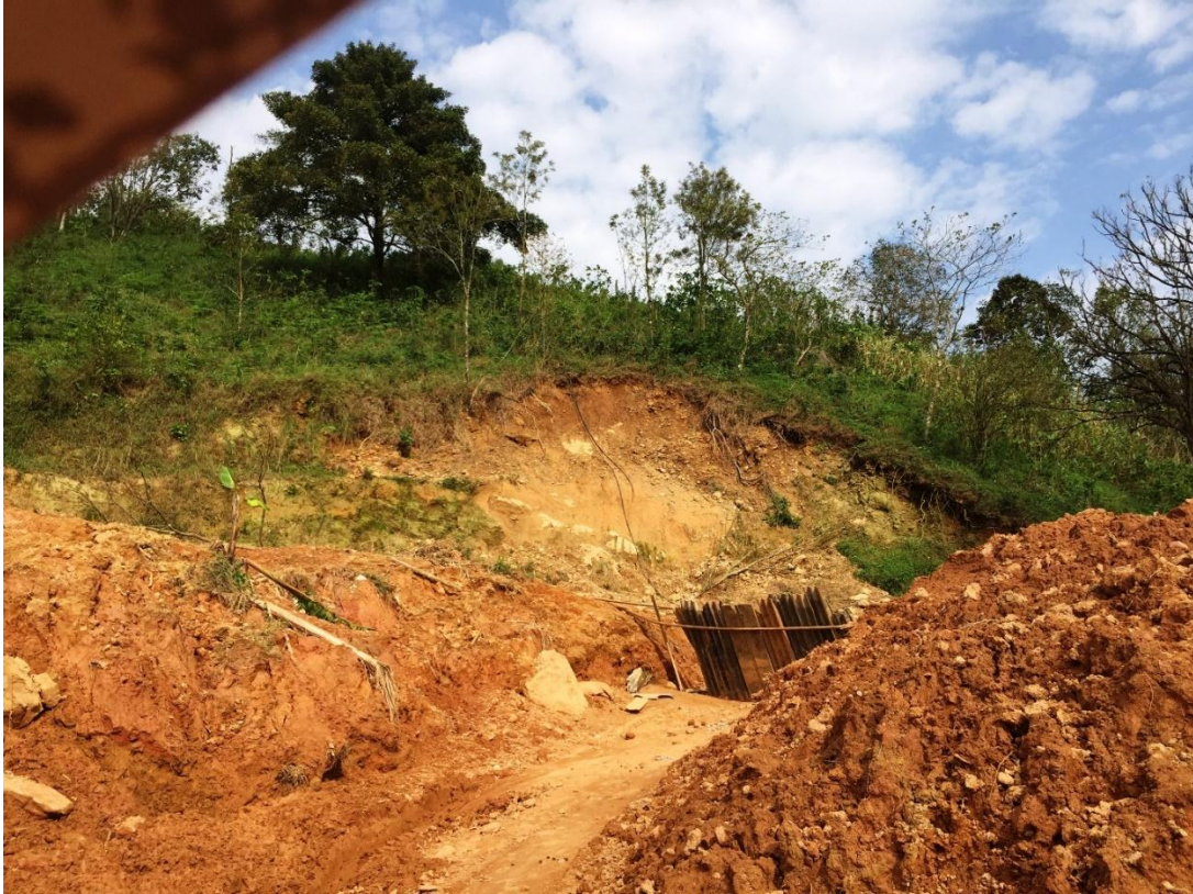
Plate 9: Slump at Nayadampoyil
