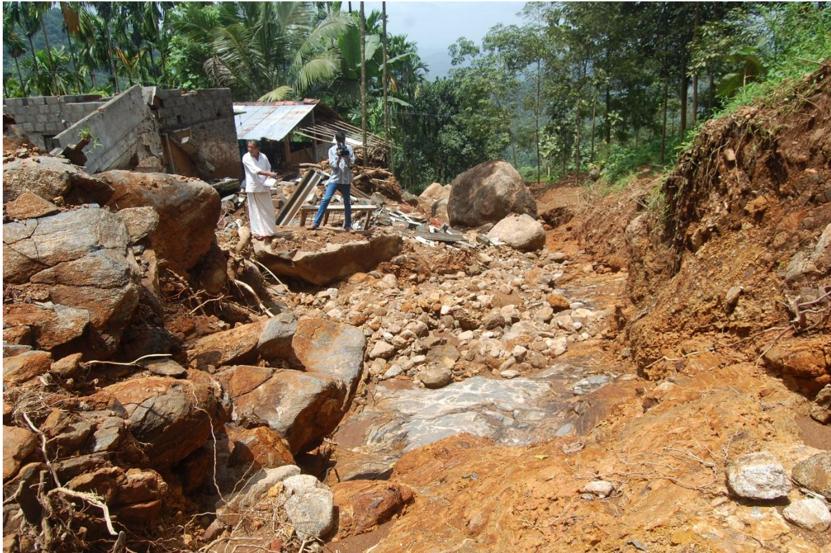
Plate 5. Plate House collapsed due to the impact of debris flow at Tharippapoyil
