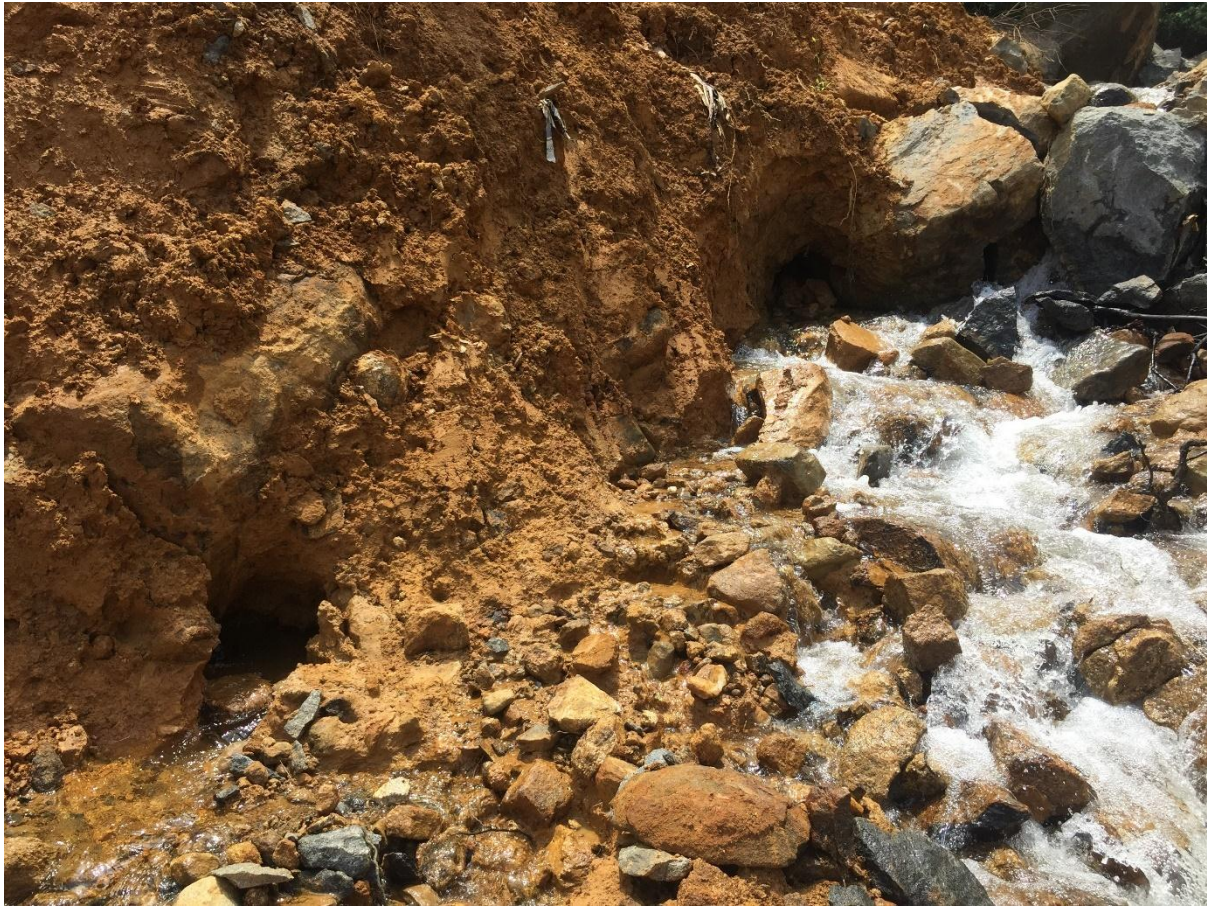
Plate 1: Sub surface tunnel erosion (Soil piping)
