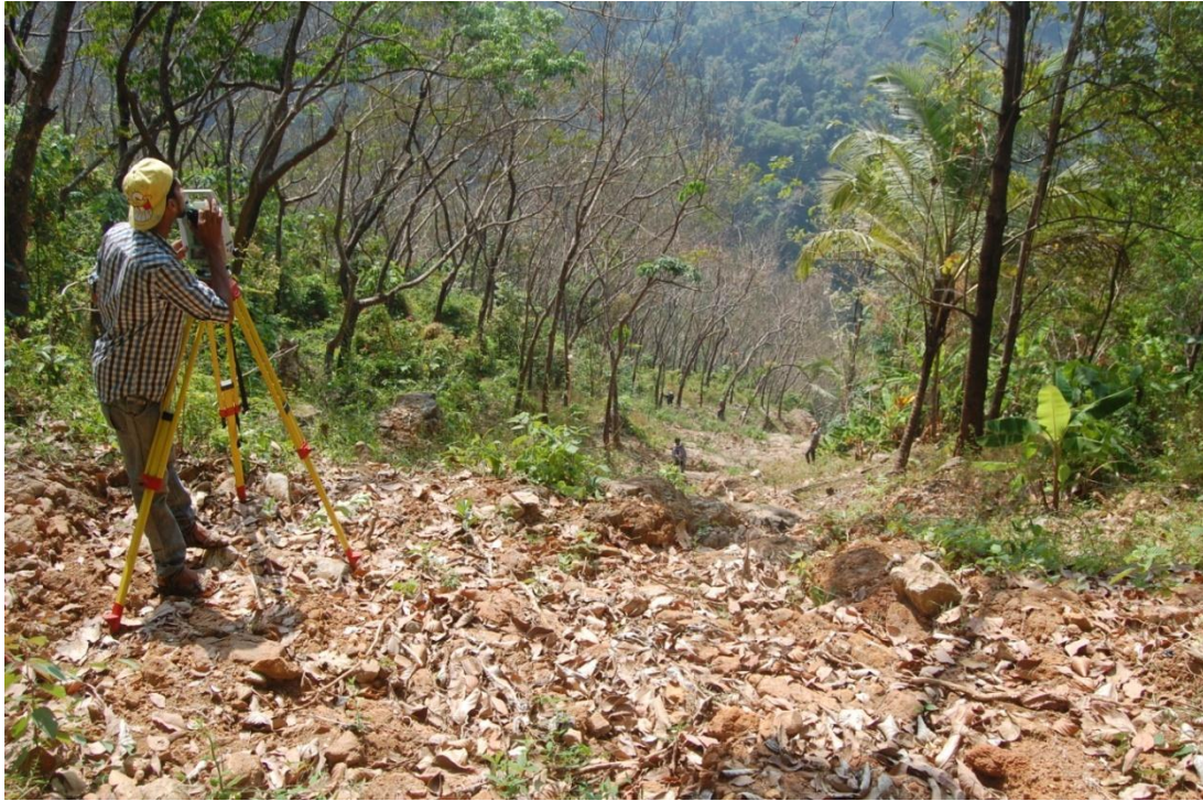
Plate 2. Survey using Total station
