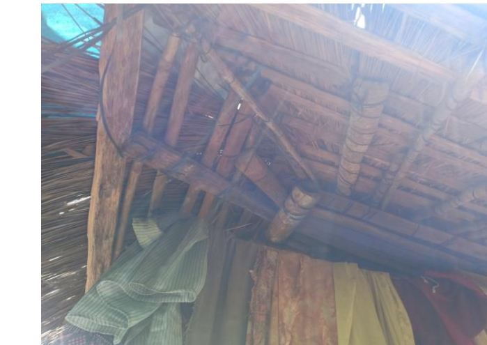
Bamboo Ridge and rafters
