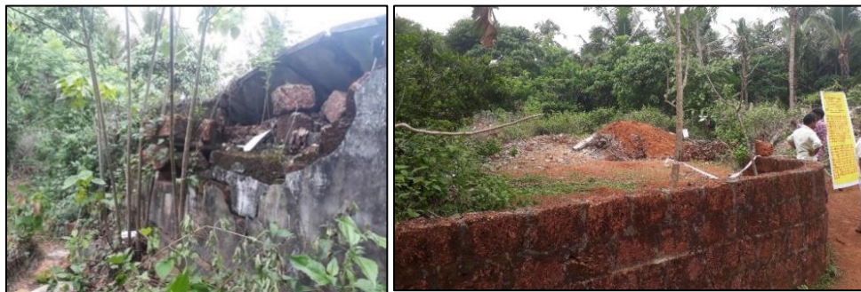
Figure 4.50: Totally damaged house of Mr. Zainuddin (2018)
