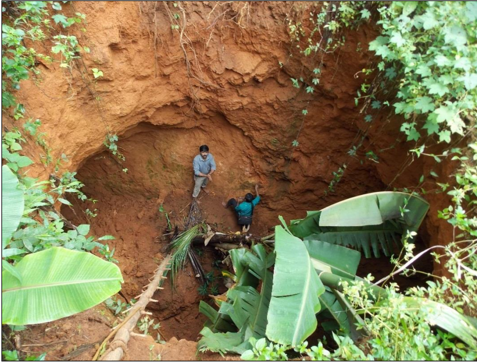
Fig 1.4 Land subsidence occurred due to piping
