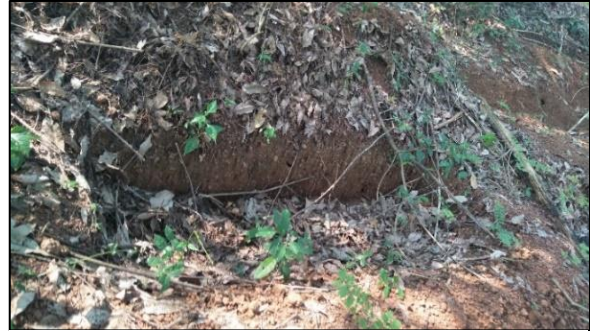
Figure. 4.8: Trenches (Mazha kuzhi) made for rainwater harvesting in the rubber plantations, which facilitate percolation of water leading to the collapse of lands.
