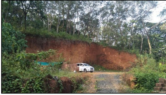
Figure 4.10: Collapsed roof of the tunnel along the road side
