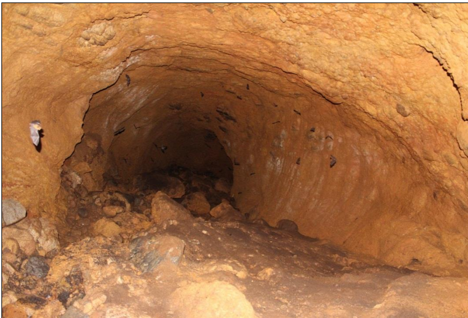
Fig 1.5 Soil pipe formed at Kottathalachi Mala
