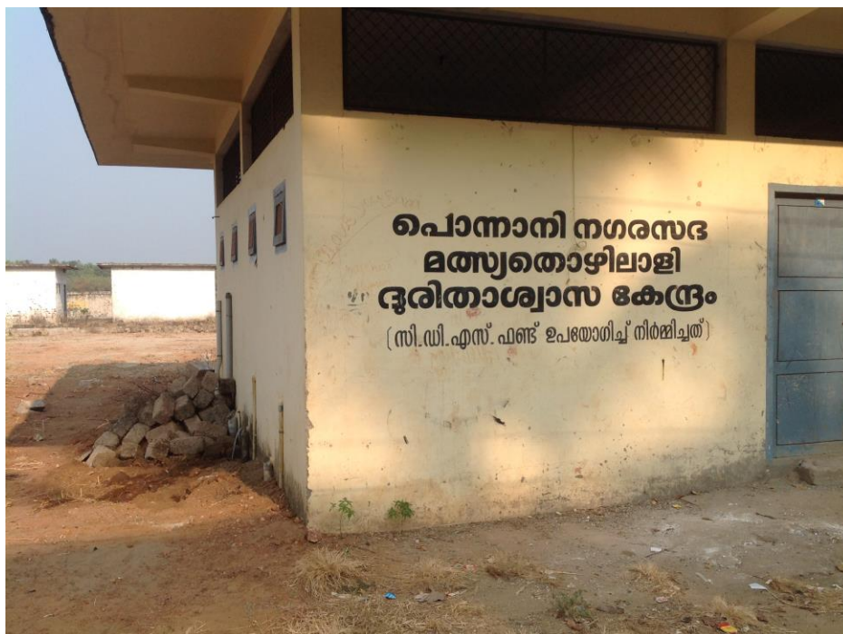
1.View of site at Ponanni Nagaram. Existing shelter in the site can be seen.
